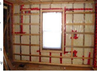
installation. It incorporates limited resistance to punctures and tears. Any penetrations, such as for an electrical junction box, must be taped and sealed in order to form an effective barrier.
